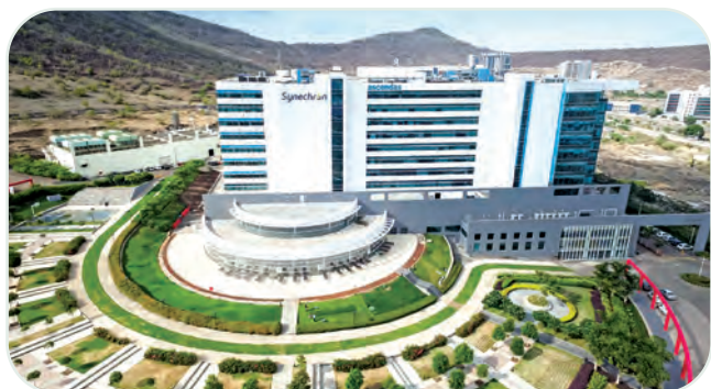
International Tech Park Pune – Hinjawadi (ITPP-H)
