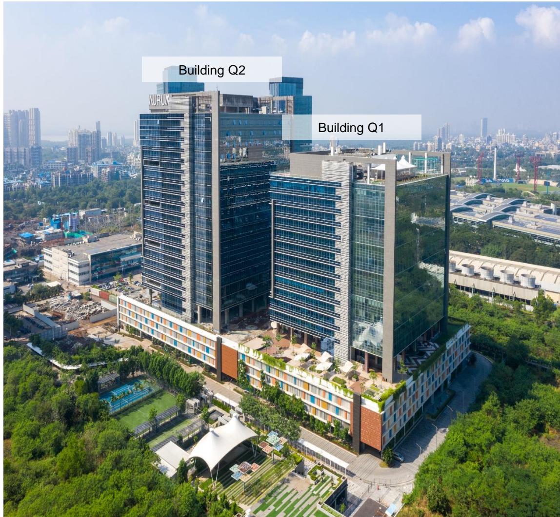
Building Q2 (left) and Building Q1 (right)
