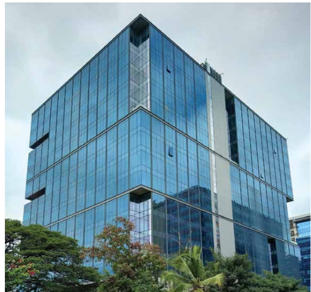
Anchor Annex building, ITPB
